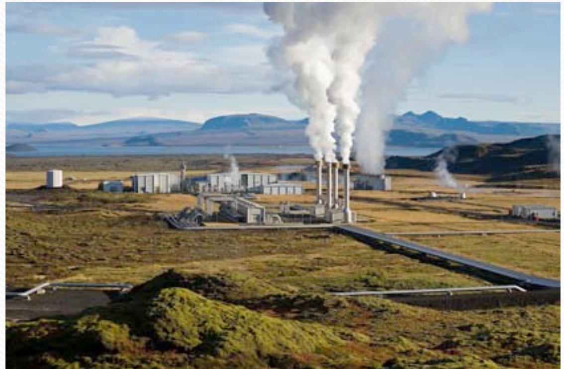
Nesjavellir Geothermal Power Plant, Iceland
