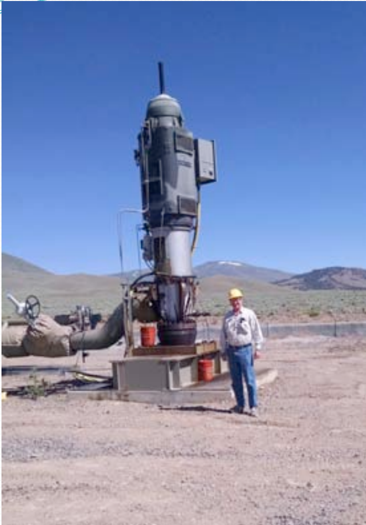
Production well @ 3000 GPM
